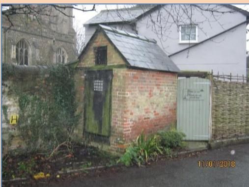
This small lock-up is next to, but not part of, the parish churchyard wall. Built in the late 18<sup>th</sup> or early 19<sup>th</sup> century, it has a slate roof and a large ventilation hole above the door. It was restored in 1977 but is now looking rather neglected.
