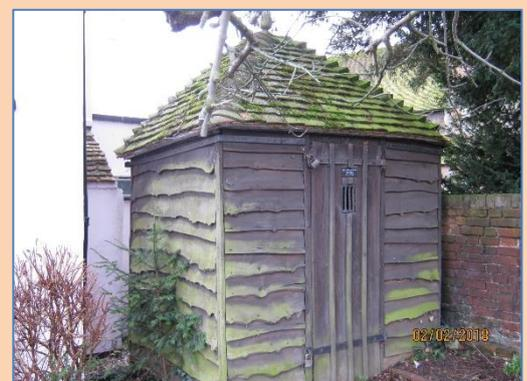
clearly much renewed since then, it has a pyramid-shaped clay tile roof and a small ventilation grille in the door. A display panel alongside gives a note on its history.
